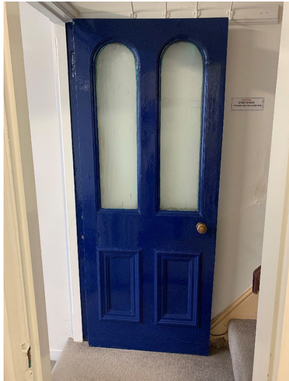
Existing door – thought to have been the original front door, prior to shop front conversion.
