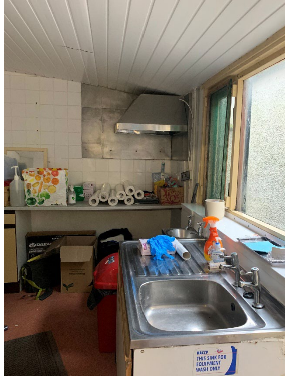
Existing kitchen in ground floor extension, to be demolished
