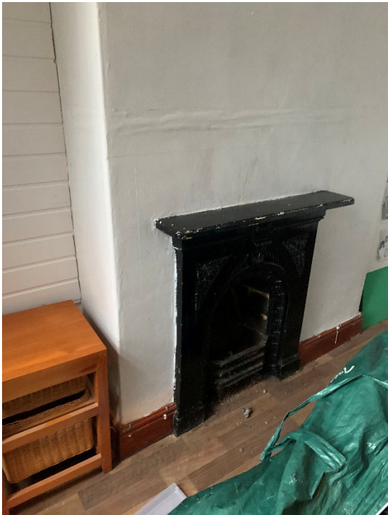
Existing first floor room
