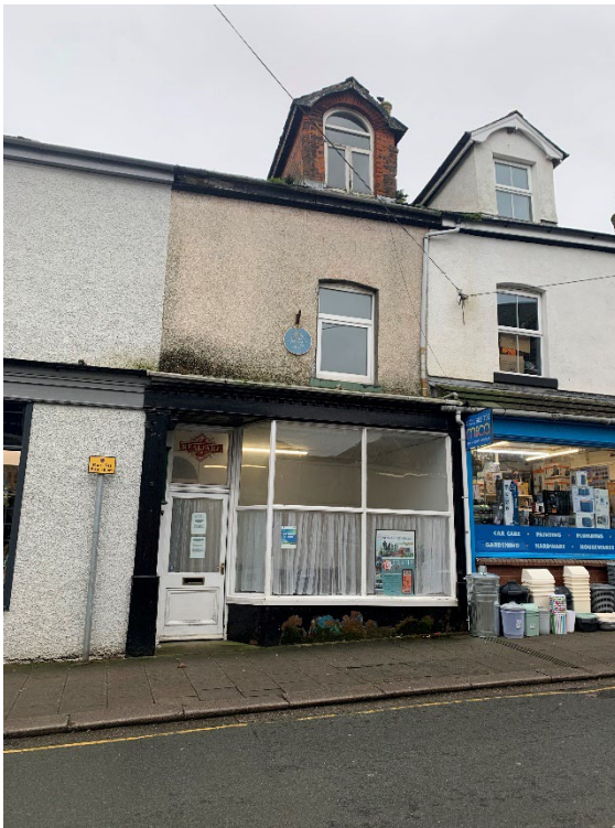
Principal Elevation prior to restoration works
