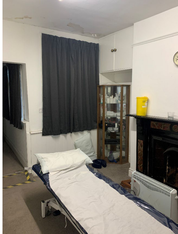
Existing ground floor room
