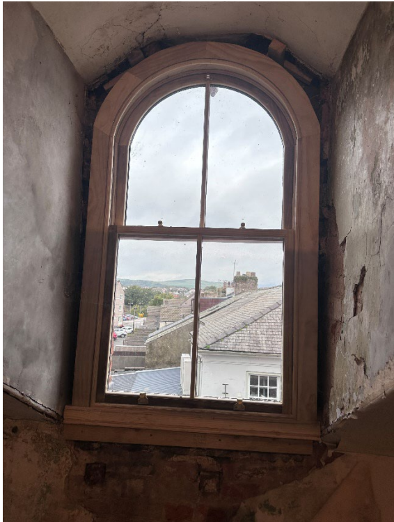
Internal view of dormer window at first floor bedroom - Norman Nicholson's former bedroom.
