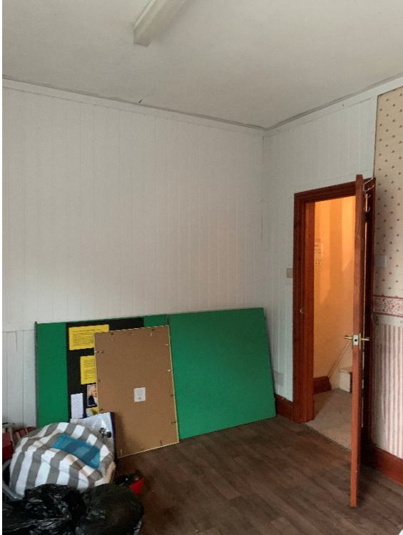
Existing first floor room
