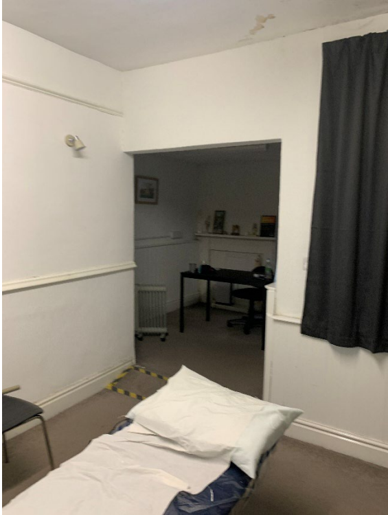
Existing ground floor room
