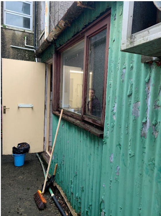
Corrugated out-shut to be removed
