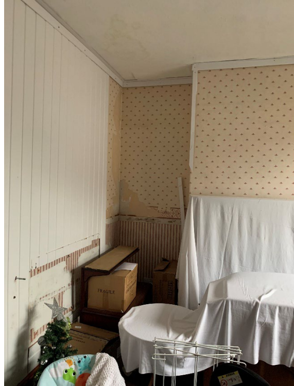
Existing first floor room
