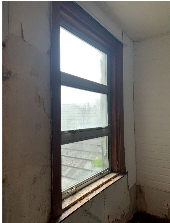
Existing first floor room
