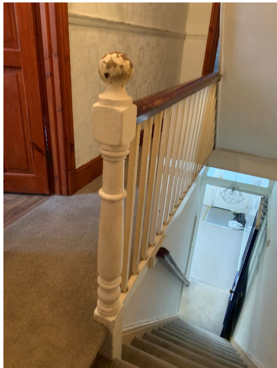
Existing staircase & balustrade
