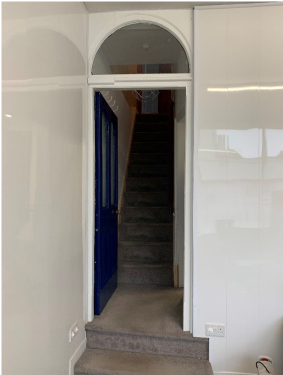
Existing door opening – formerly the division between the shop and living accommodation
